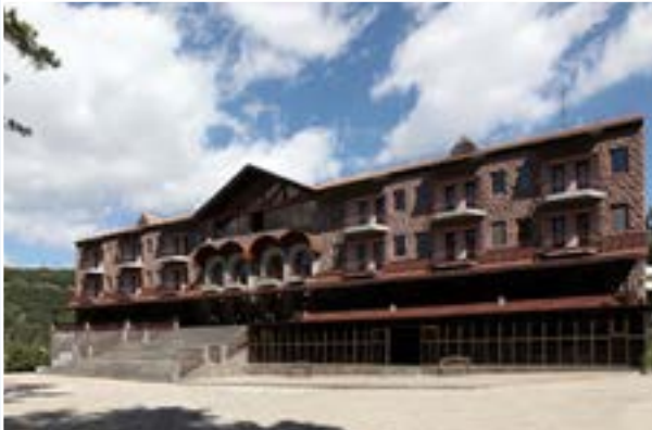
Training Centre of the Central Bank of the Republic of Armenia (Tsakhkadzor)
