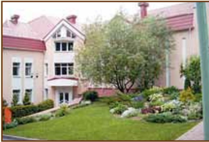
Training Centre of the National Bank of the Republic of Belarus, Village of Raubichi
