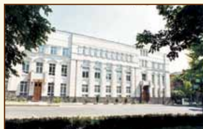
Central Bank of the Republic of Armenia Main Building
