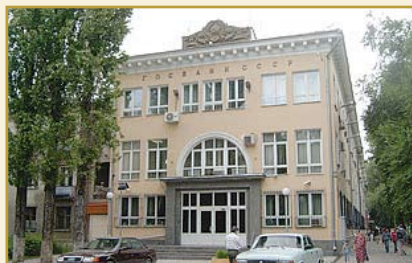
National Bank of the Kyrgyz Republic Main Building
