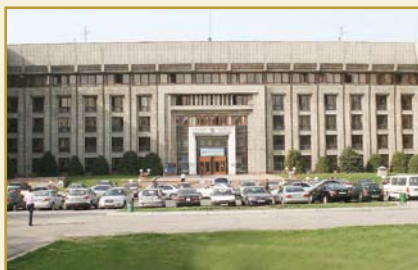
The Agency of the Republic of Kazakhstan on regulation and supervision of financial market and financial organizations Main Building
