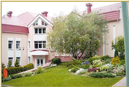
Training Centre of the National Bank of the Republic of Belarus, Village of Raubichi
