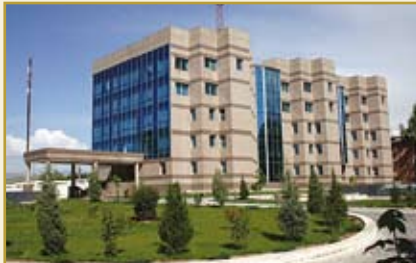
National Bank of Tajikistan Main Building
