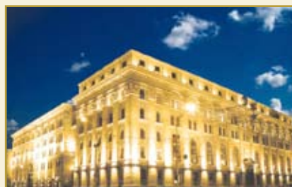
National Bank of the Republic of Belarus Main Building
