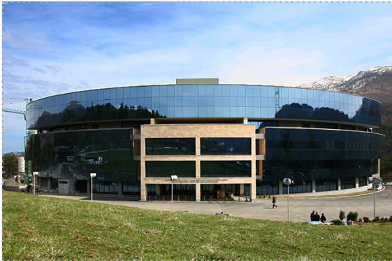
Training and Research Centre of the Central Bank of Armenia (Dilijan)
