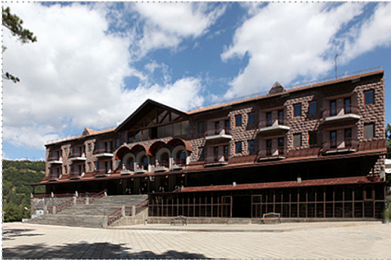
Training Centre of the Central Bank of Armenia (Tsakhkadzor)
